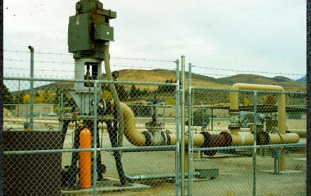
The second major requirement for pumps stems from the need to pump the working fluid through the heat exchangers and to the turbine inlet. The pumps are usually multi-stage, vertical canned pumps.
