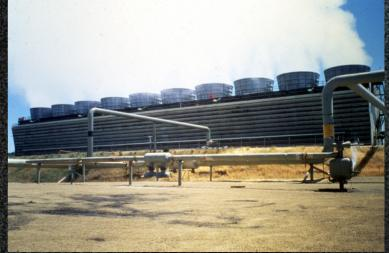
Adding enhanced evaporation cooling to air condensers can improve summer efficiency by as much as 40+%, greatly improving the economics of such operations.
