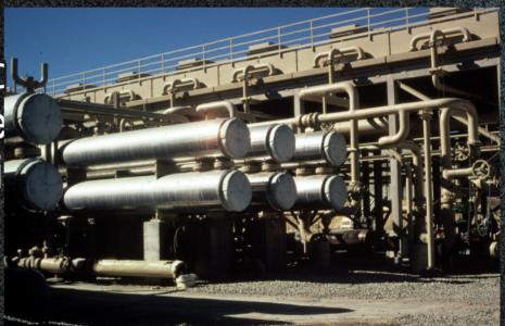
Another major cost that is specific to the binary cycle is the number of pumps required and the significant parasitic load they place on the plant. Because brine from a liquid-dominated reservoir should be maintained as a single-phase flow through the heat exchanger, production well pumps are used.
