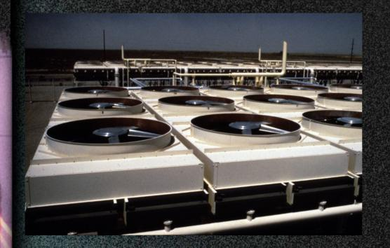
The best of both systems may be the hybrid based on the use of air coolers but with injection of a water mist into the airflow of the air cooler or the spraying of water onto fibrous material used to enclose the walls of the cooling tower. This can significantly increase cycle efficiency and output during peak demand periods in a summer peaking area.
