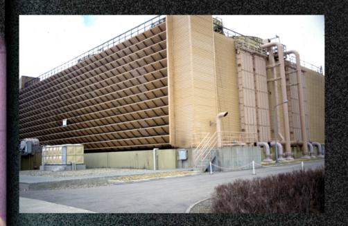
A water-cooled cycle capable of approaching the wet bulb temperature presents a significant advantage, as far as overall power generation is concerned, in comparison to a dry cooled binary cycle that approaches the dry bulb instead of the wet bulb.
