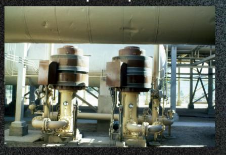
In addition to the additional capital cost attributable to the need for production and/or working fluid circulating pumps, pumping requirements result in a parasitic load of 10 to 15% of the power that is generated, a significant reduction in the amount of power that is available for sale.
